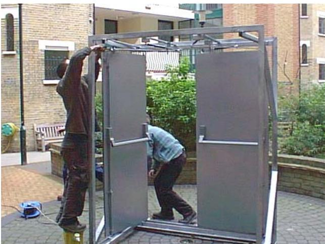
The prototype is based on simple draw back doors
