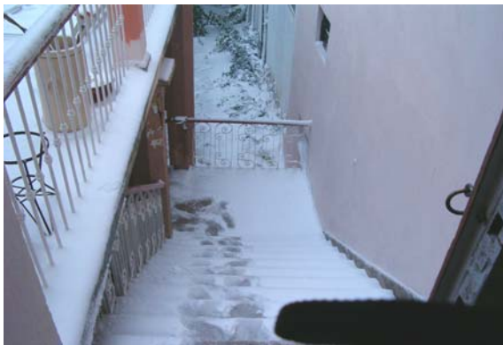
The subway is now used, even in winter
