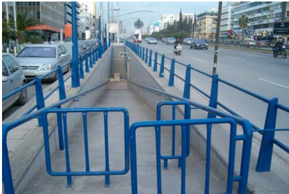
Gates to stop access by motor cyclists – but difficult for disabled to access subway
